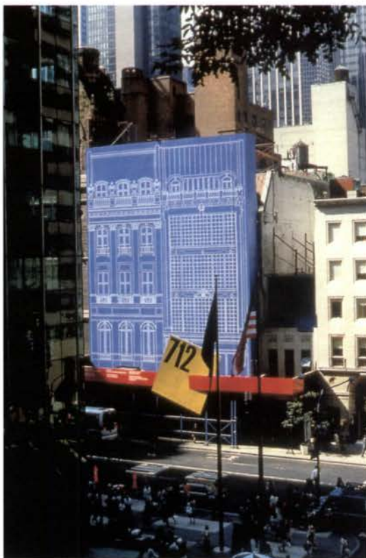
712 Fifth Avenue, New York, 1987. Construction Sites.
